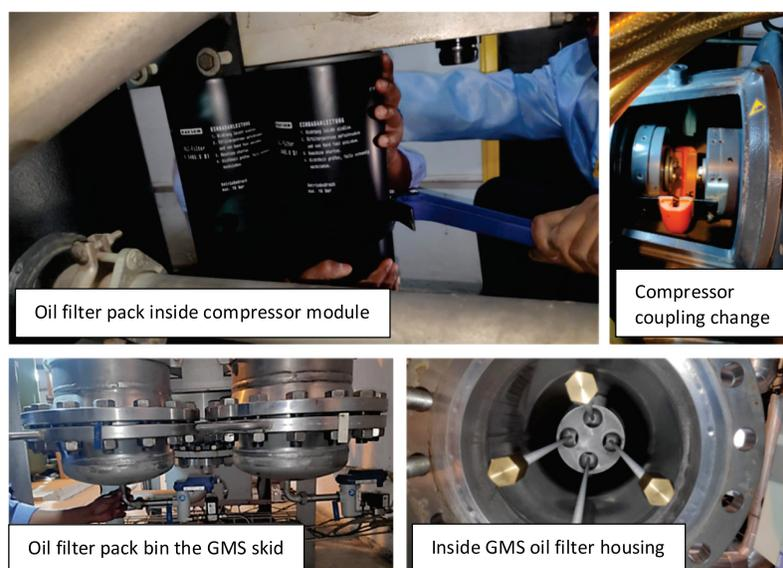
Fig. 3.1.2.1 Various components of the compressor and the GMS of the helium refrigerator .
