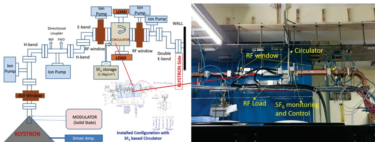
Figure 2. Installation of  $\text{SF}_6$  gas-based Isolator for protection against reflected power.
