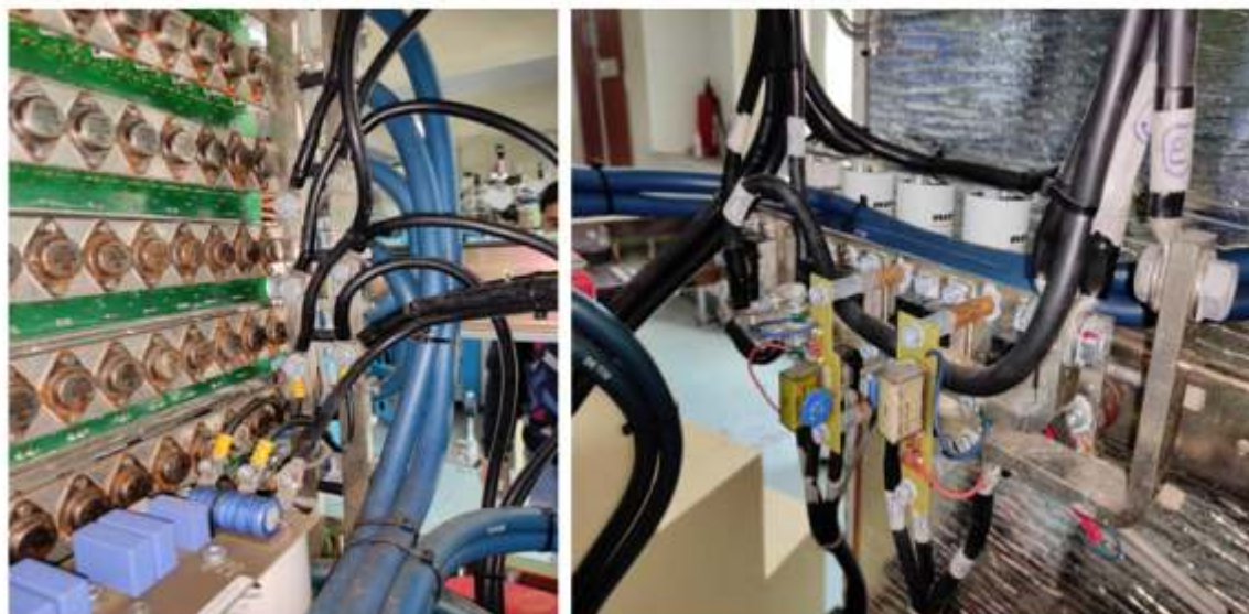
Fig 3: Rusting on the electronic components and chassis of the magnet power supply and magnetic steer/scanner installed in the beam line.
