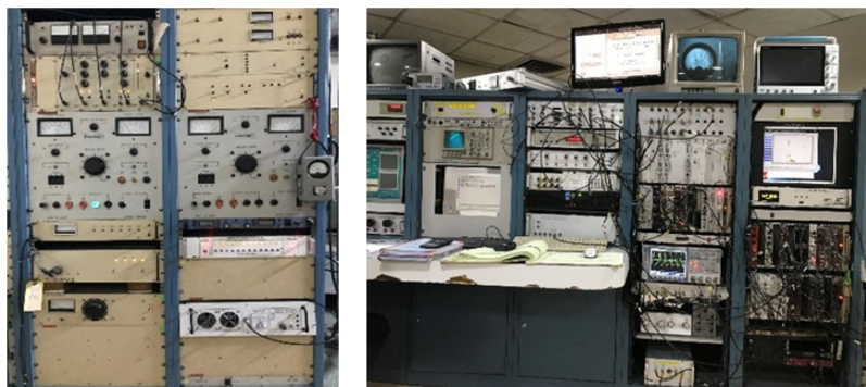
Figure 3.15: Pelletron beam pulsing system electronics with multi-level fault detection system.
