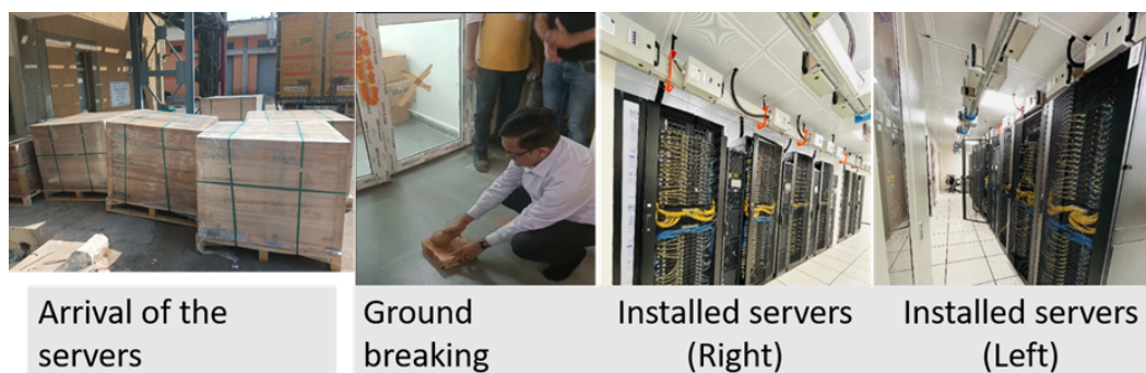
Figure 3.21: Photographs of different stages of the data centre.
