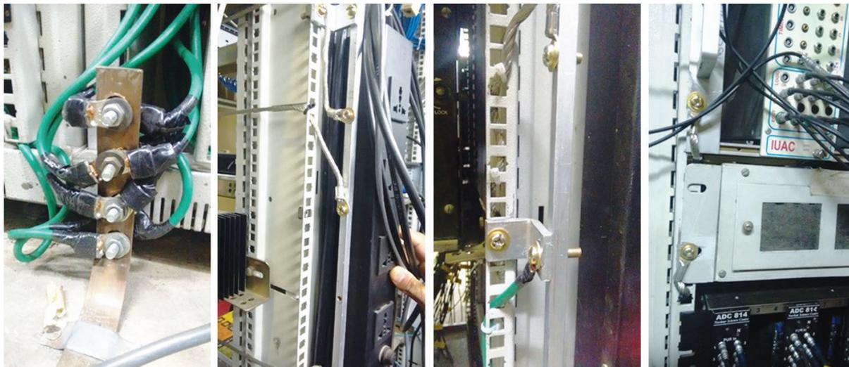
Fig. 4.2.2: Clean ground connections for INGA racks, crates and NIM bins.
