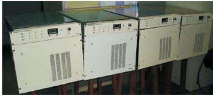
**Fig. 5. High current scanner magnet power supplies**
