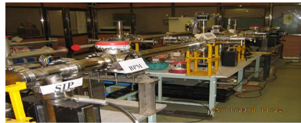
Fig -2. Mock assembly of new TL-1.
