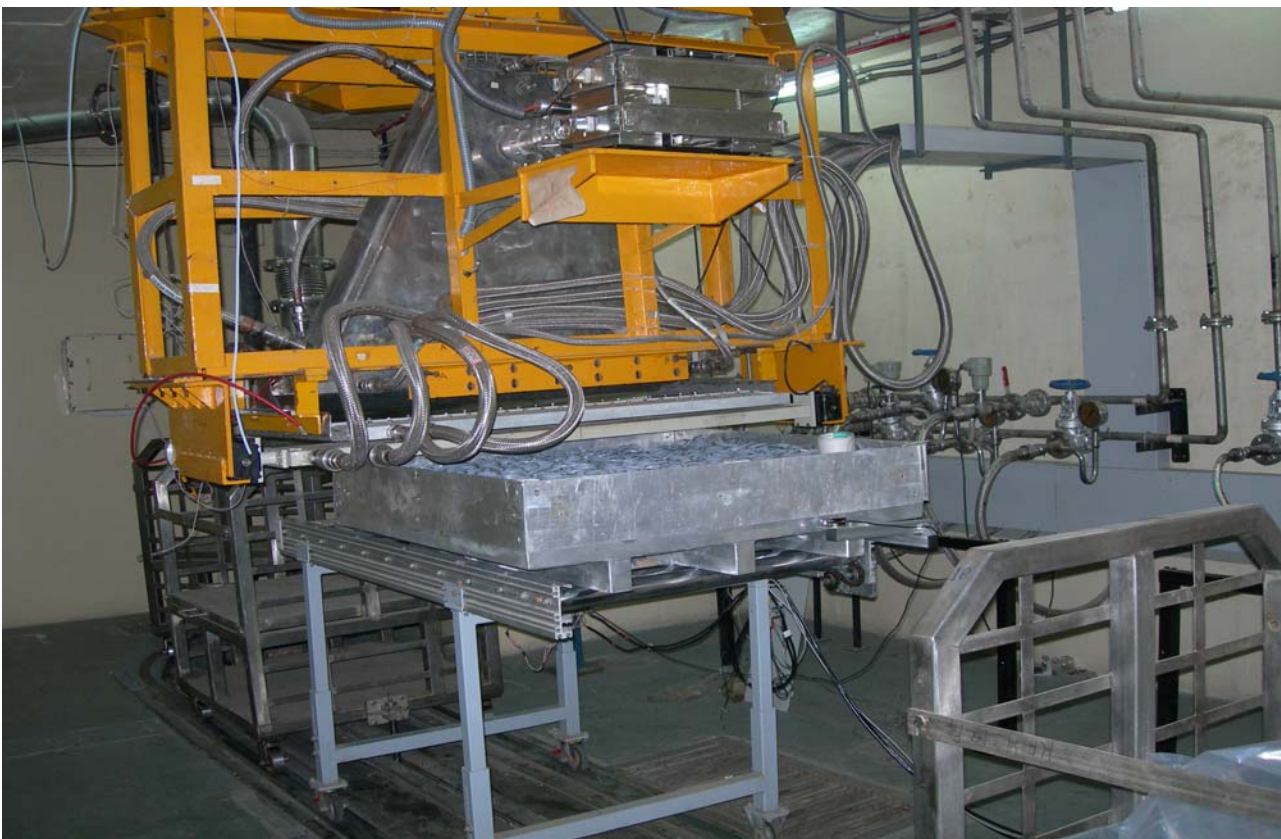
Figure 1: To and Fro Conveyor System, showing radiation tray filled with polyethylene gaskets to be irradiated, also seen the limit switches, the stepper motor below the trolley, the scan horn of Linac and water cooling lines of scan horn
